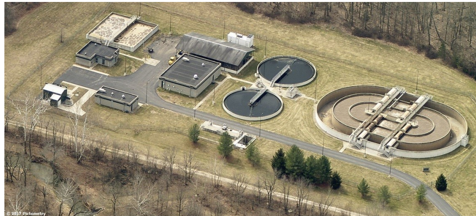
Ellettsville Wastewater Treatment Plant
